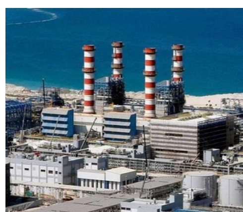
JEBEL ALI POWER AND DESALINATION STATION "M" - DUBAI
