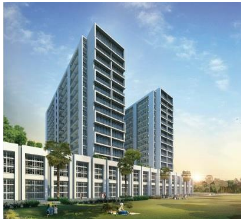
TOWER A OF NAVITAS (G+15 BUILDINGS) AT AKOYA OXYGEN ON PLOT NO. X-MU-B3, AL YUFRAH 2 - DUBAI
