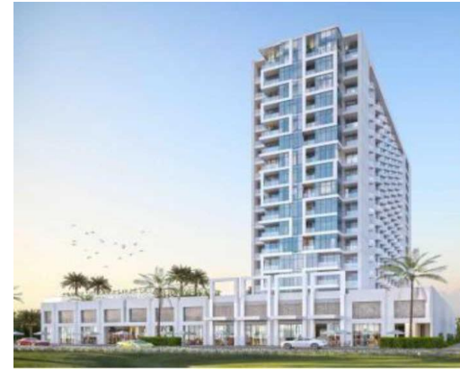
TOWER E OF NAVITAS AT AKOYA OXYGEN ON PLOT NO. AO.MU.002 AL YUFRAH 2 - DUBAI
