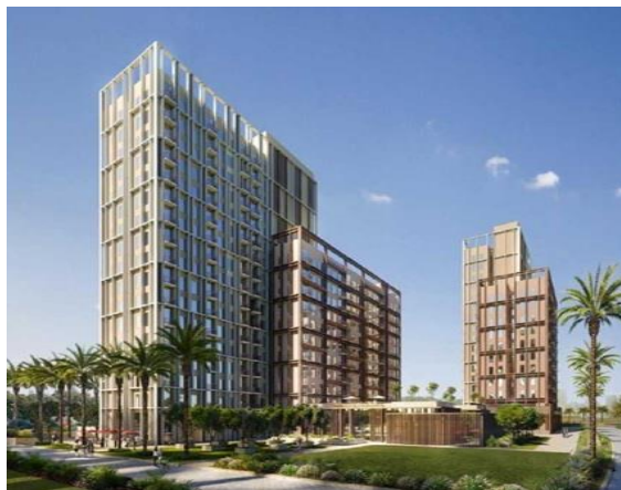
COLLECTIVE 1 (B+G+16+M) RESIDENTIAL TOWER ON PLOT NO. 20.0004 AT DUBAI HILLS ESTATE - DUBAI
