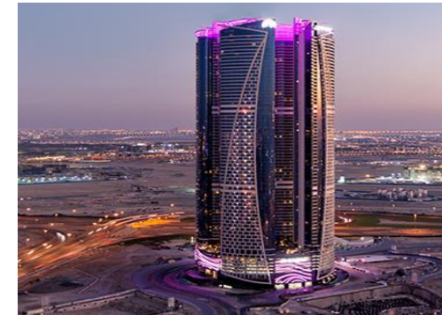
PARAMOUNT TOWER BY DAMAC - DUBAI (2) ESCALATORS ONLY
