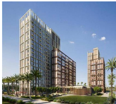
COLLECTIVE 2 (B+G+M+18+R) RESIDENTIAL TOWER ON PLOT NO. 6311119 AT DUBAI HILLS ESTATE - DUBAI
