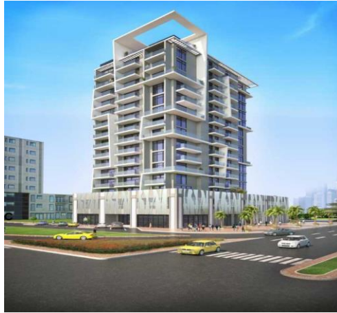
2B+G+P+ROOF FLOOR RESIDENTIAL BUILDING ON PLOT NO. AFMU 004B AT AL FURJAN - DUBAI
