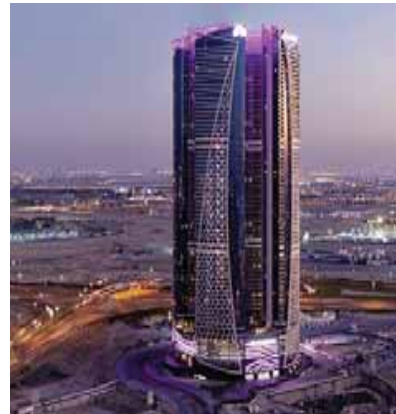
PARAMOUNT TOWER BY DAMAC - DUBAI (2) ESCALATORS ONLY
