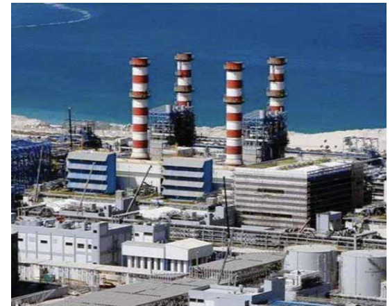
JEBEL ALI POWER AND DESALINATION STATION "M" - DUBAI
