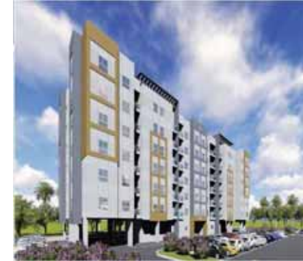
R1083 AL QUSAIS RESIDENTIAL DEVELOPMENT (19 BUILDINGS) - DUBAI
