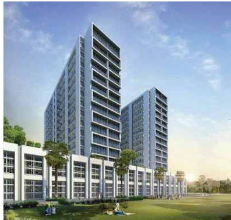
TOWER A OF NAVITAS (G+15 BUILDINGS) AT AKOYA OXYGEN ON PLOT NO. X-MU-B3, AL YUFRAH 2 - DUBAI
