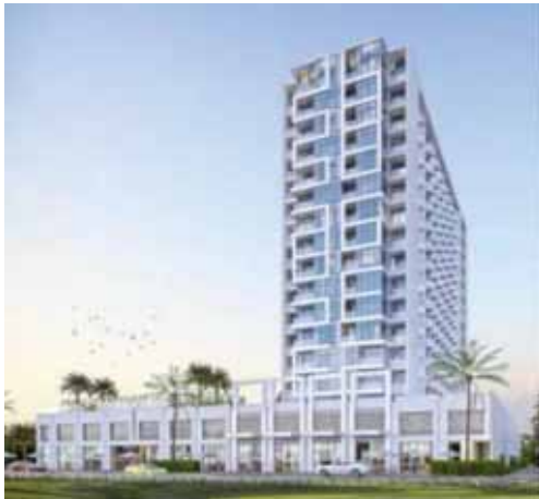
TOWER E OF NAVITAS AT AKOYA OXYGEN ON PLOT NO. AO.MU.002 AL YUFRAH 2 - DUBAI
