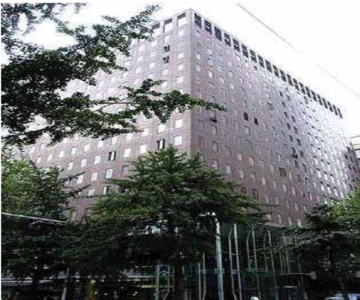
KOLON BUILDING SEOUL, KOREA
